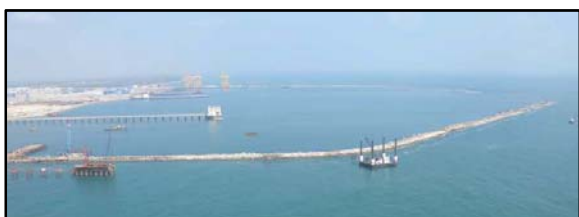
Aerial View Kattupalli Port
